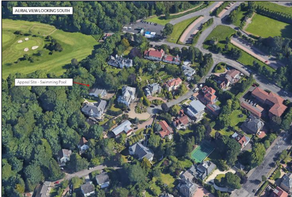
Figure 8: Aerial view of the appeal site looking south.
