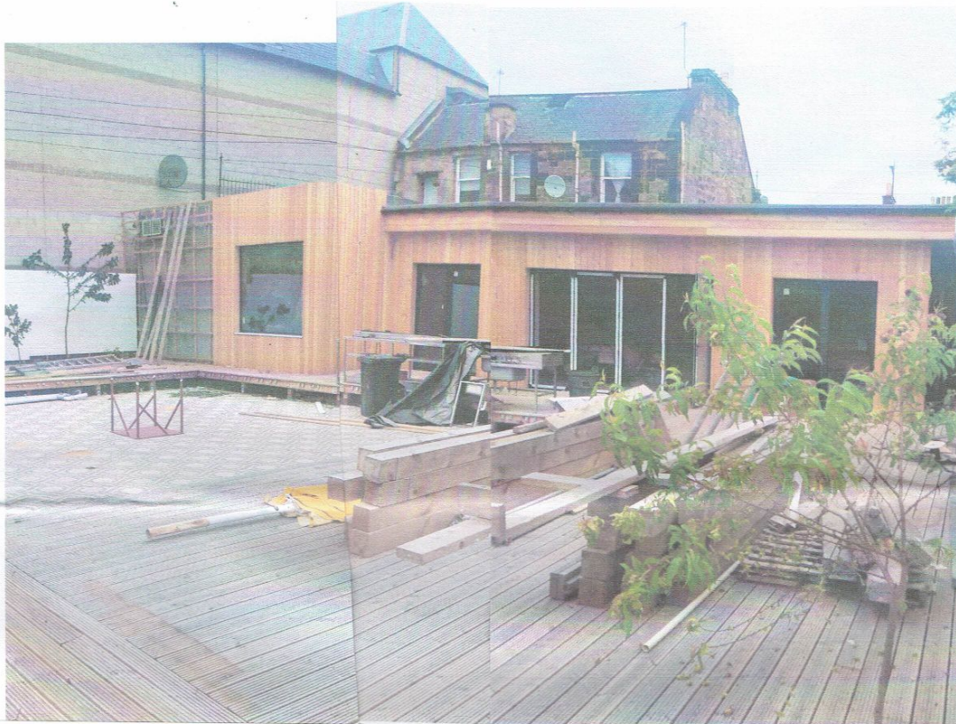
PHOTOGRAPH OF REAR ELEVATION & GARDEN UNDER CONSTRUCTION
