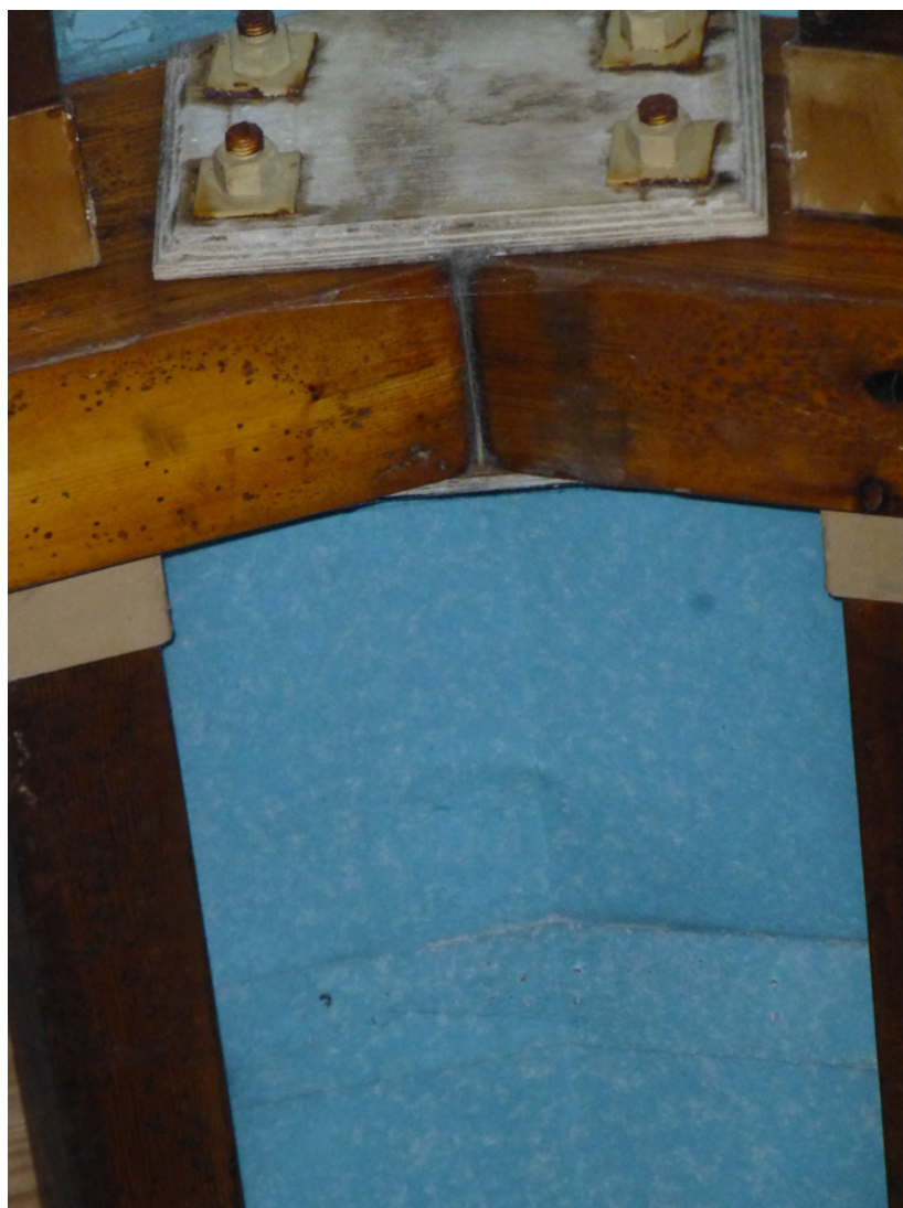
Glulam Portal Frame Apex Connection Detail
