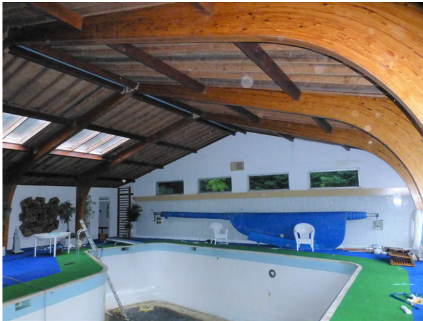
Glulam Frames looking South
