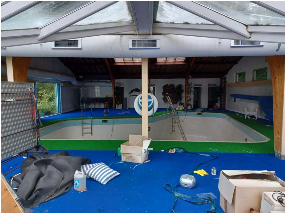
Figure 6 – Internal view of swimming pool looking East.
