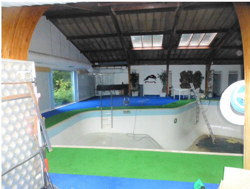
Glulam Frames Looking East
