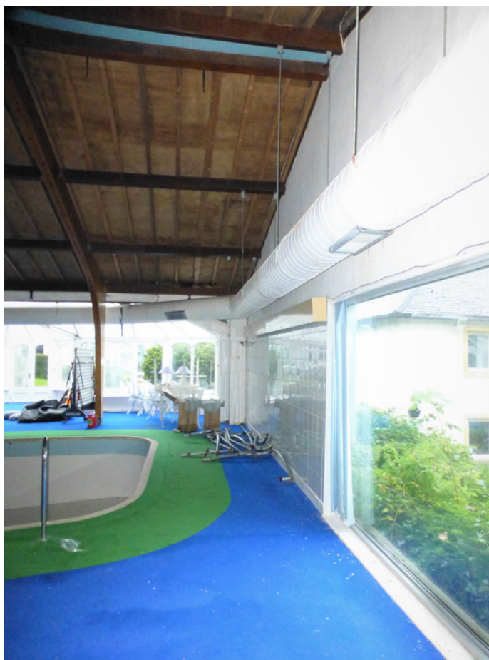
Glulam Frame looking West
