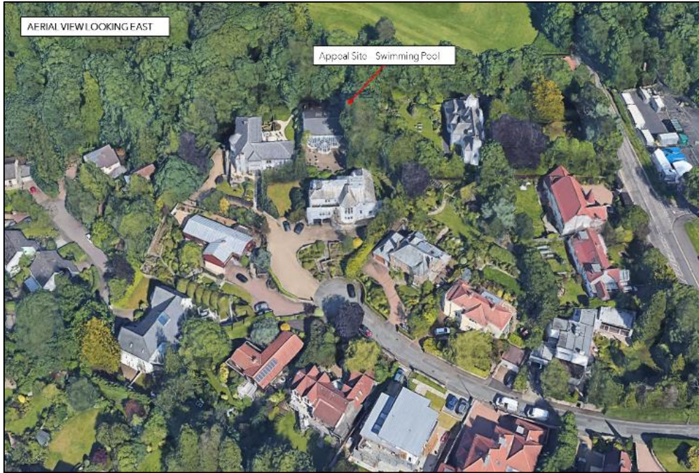
Figure 6: Aerial view of the appeal site looking east.
