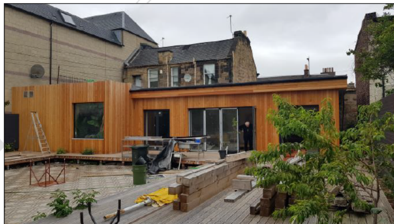
Fig 13 - view from rear garden showing the upstairs residential flat with a chimney stack on its gable elevation through which the kitchen flue will extract
