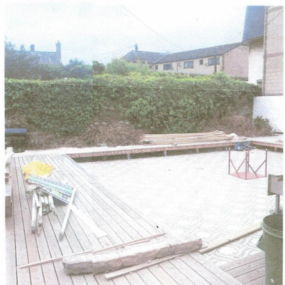
PHOTOGRAPH OF GARDEN UNDER CONSTRUCTION & SOUTH GARDEN WALL
