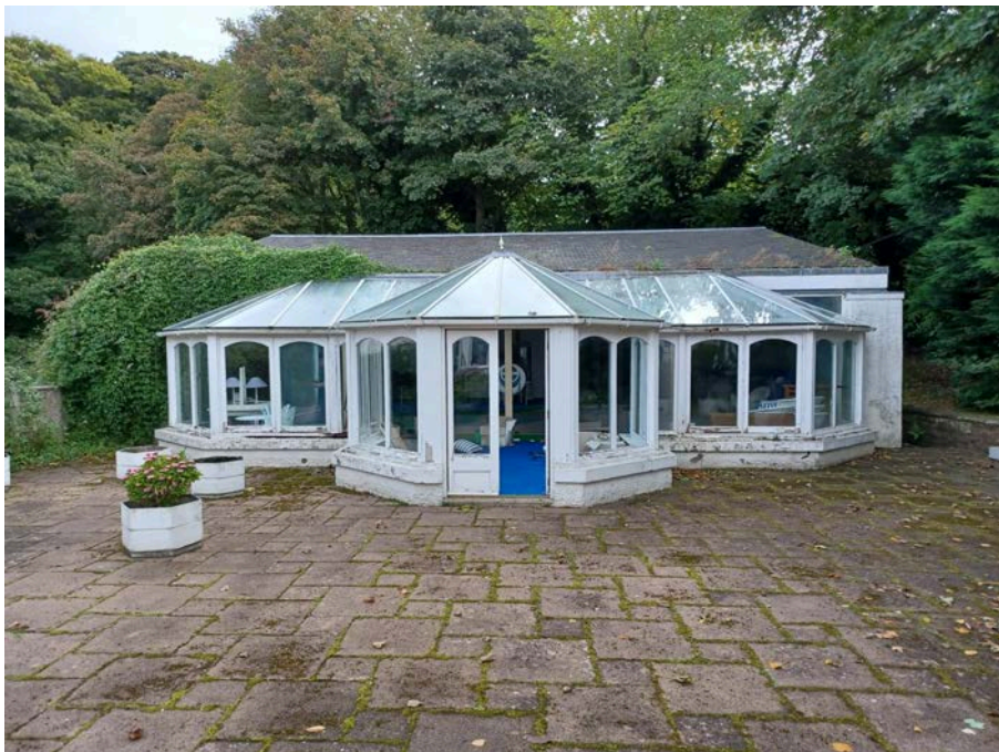
Figure 7 – view of 2007 conservatory added to front of portal frame.
