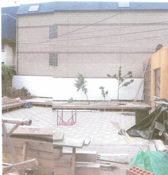
PHOTOGRAPH OF GABLE OF BUILDING TO THE EAST
